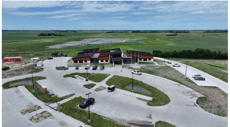
CPNRD's new office and education center is nearing completion. Staff plans to relocate to the facility in late fall.
