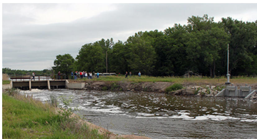
Thirty Mile Canal headgates in Dawson County
